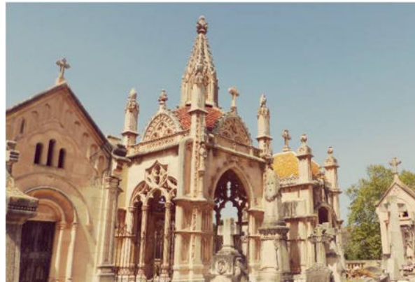
4. CEMENTIRI MUNICIPAL Reforma de Gaspar Bennazar, 1938
